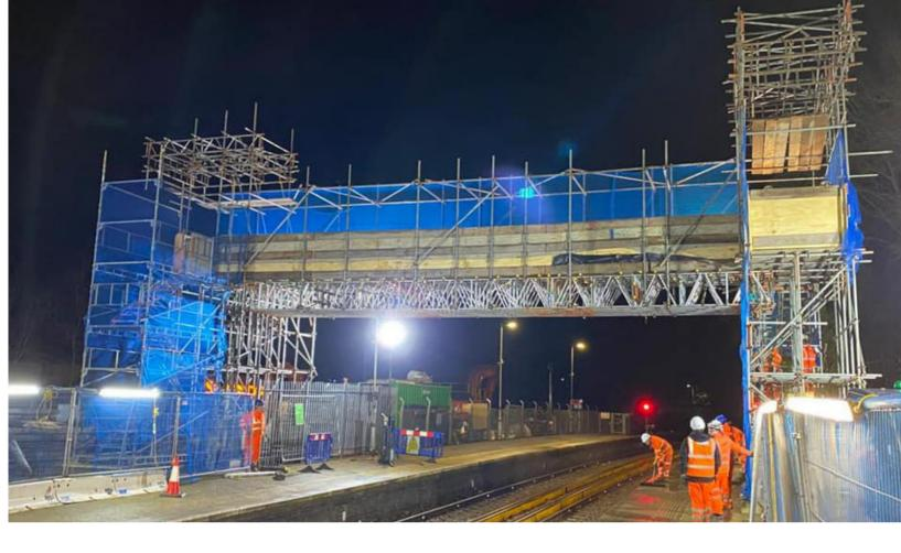
What made this rail scaffolding project so unique was that the bridge span was built at ground level and lifted in place using a 50T during a 27-hour long abnormal possession. The scaffold was also erected in two separate phases, with a mixture of both normal daytime working and weekend/possession working.
