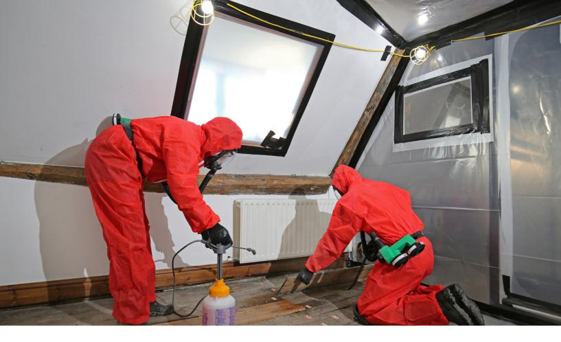
To mitigate this, the enclosures were split into manageable sizes and operative numbers were kept to a minimum. We adopted a systematic approach, removing small areas at a time and replacing them, before moving on to the next area. Crawl boards were also used, where needed.
