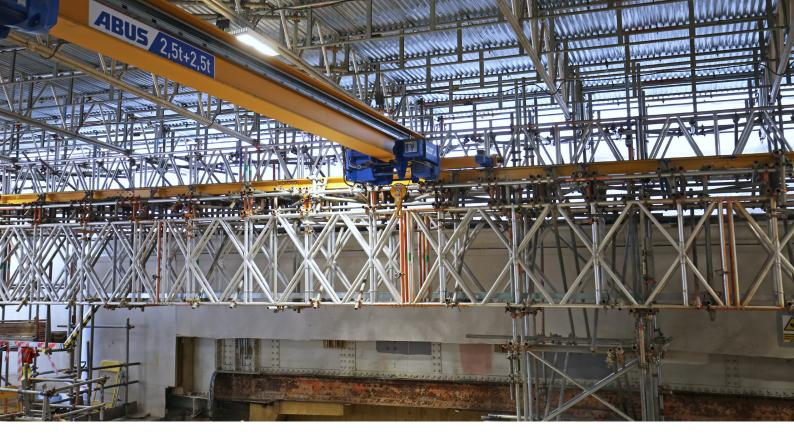
process, including fall protection systems, regular inspections, and adherence to SG4:15 and TG20:21.
