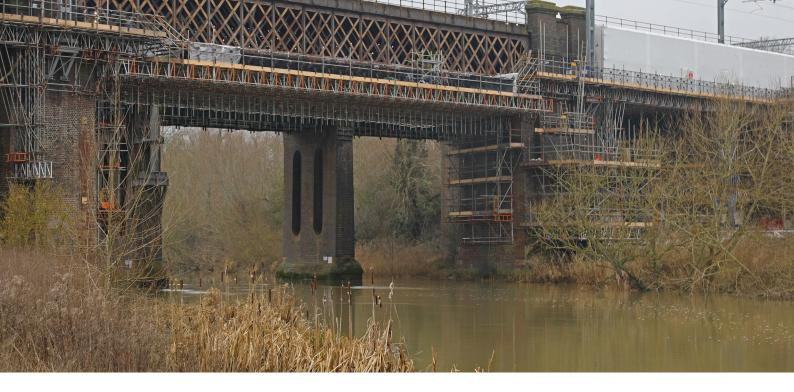
components to support both internal and external bridging beams. These support systems also facilitated temporary access for scaffold operatives during the installation process. We are working closely with BAM and ARUP to navigate the challenges posed by structurally unsound areas of the piers, ensuring our solutions meet all safety requirements throughout.
