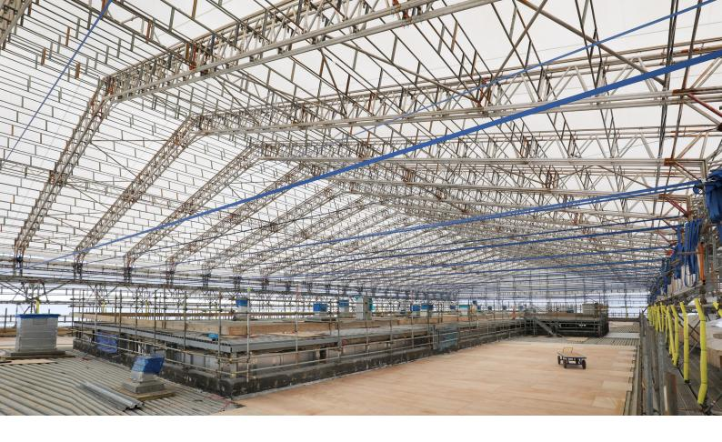
Designed in-house by Jak Patterson-Fields, it was built in 6.4-metre-wide sections at ground level, craned into place, and rolled out toward the northern end of the site. The system, now complete and handed over, is scheduled to remain in place until dismantling begins, which will follow the same methodology in reverse, with each section lowered and safely deconstructed on the ground.
