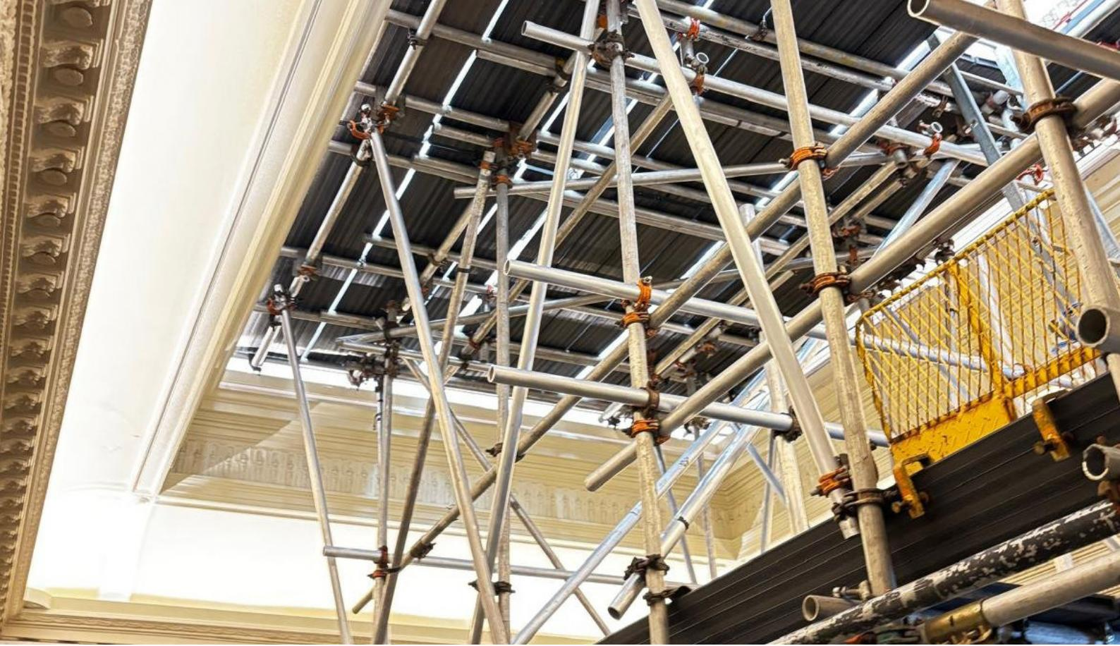
level working platforms that adapted to the architectural constraints of the stairwell and dome. Scaffold fixings were carefully positioned to avoid damage to ornate cornices, balustrades, and tiled finishes.
